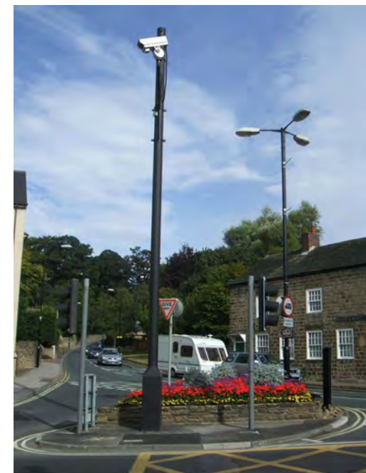
Despite bright, decorative planting this junction, unfortunately, is dominated by insensitive and intrusive highway infrastructure.
