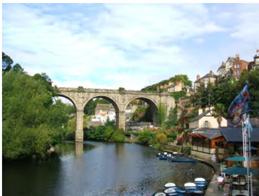
The Viaduct seen from Waterside.
