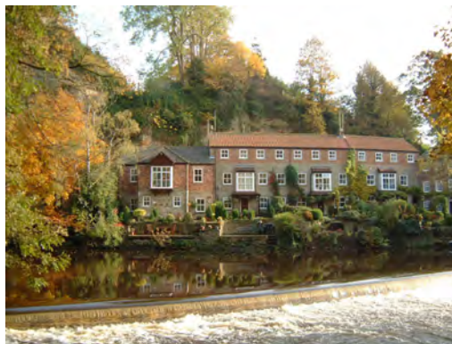
Castle Mills from across the river.
