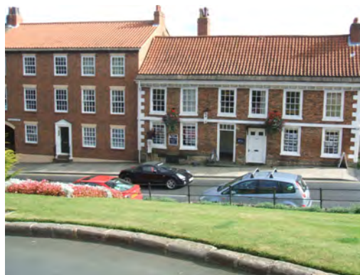
Buildings on Lower High Street seen from the elevated frontage of Knaresborough House.
