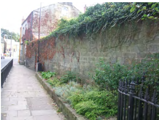
High wall adjacent the footway on Bond End.
