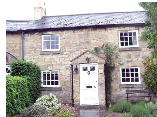
Horizontal sliding sashes.
