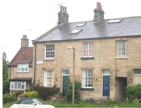
An example of ashlar limestone and rooflights.
