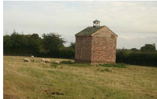
The Pigeon House, off Main Street, sits in a meadow containing the suggestion of possible footings of many, long since demolished, buildings.
