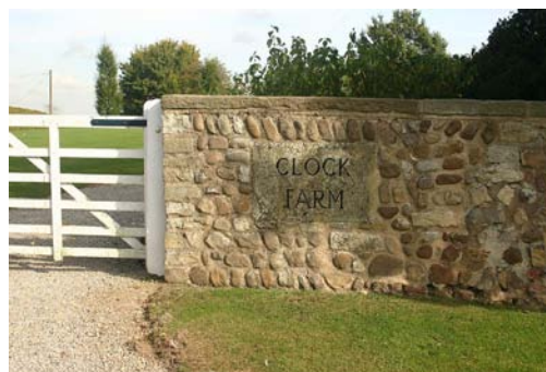
Clock Farm wall by Main Street entrance - cobble construction with flat coping stones.
