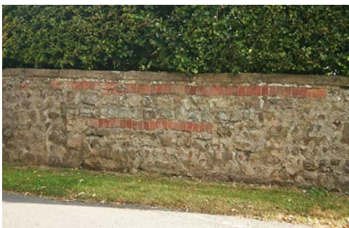
Clock Farm wall is composed of various natural and reused materials.
