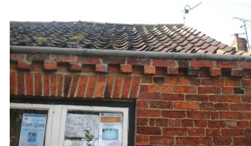
Brickwork detailing on the Post Office, Main Street
