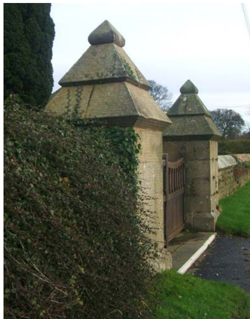
Prominent gate piers at the Church.
