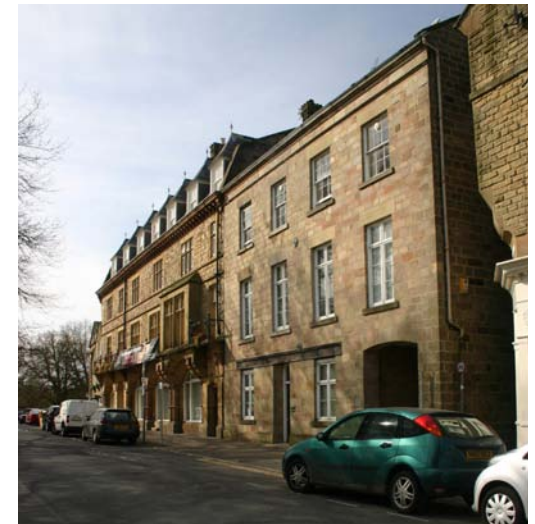
Many properties on Regent Parade front directly onto the footway.
