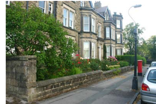
Park Avenue on the edge of The Oval.
