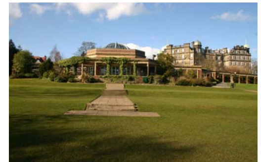
Sun Pavilion with Windsor House (Cornwall Road) behind.
