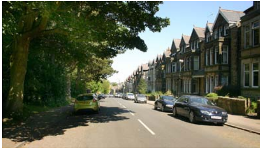
Three storey terraced properties on Harlow Moor Drive, with Valley Gardens on the left.
