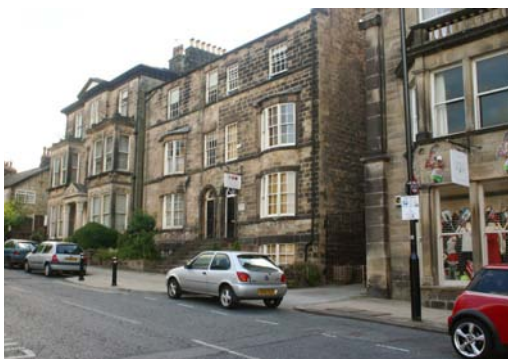
An early C19 pair with bow windows on Cold Bath Road.
