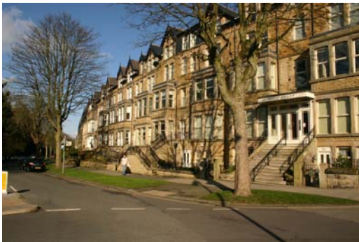
Four storey terraced buildings on Valley Drive.
