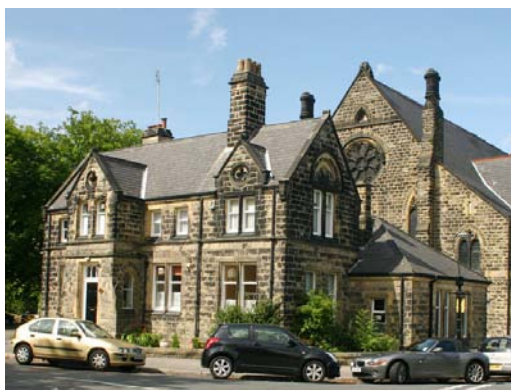
Welsh slate roof with projecting gables and robust stone detailing on this building allied to Trinity Church.
