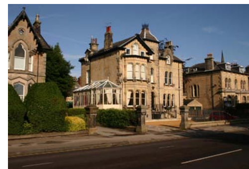
Large villas on Leeds Road.
