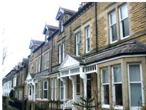
Two-paned sashes separated by stone mullions, on St Georges Road.
