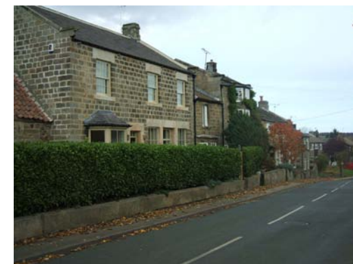
A variety of single and 2 storey bay windows.
