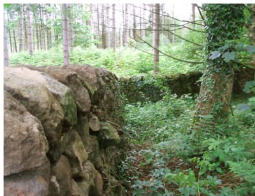
Dry stone wall alongside Ripon Rowell.
