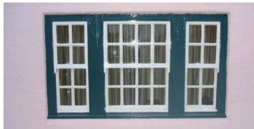
Sash windows on Garden House
