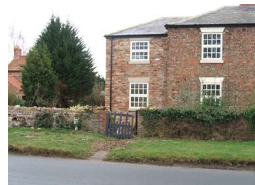
Recent extension to a traditional property in the village.
