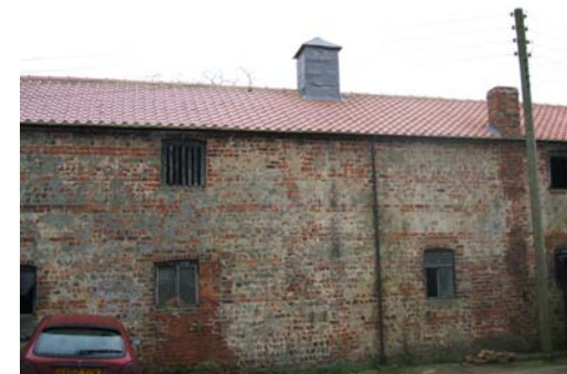
Traditional barn constructed of cobble walls with brick lacing courses.
