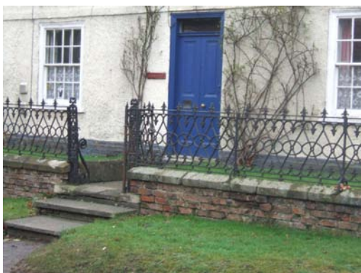
Rosecroft's distinctive railings.
