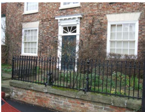
Pedimented doorway with radial fanlight above the door.
