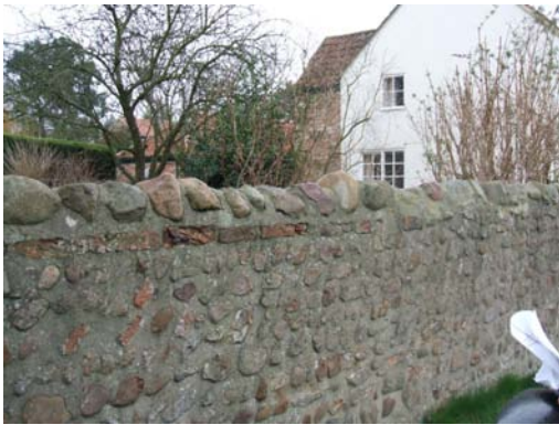
An example of cobbled walling.
