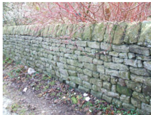
Capped dry stone wall.
