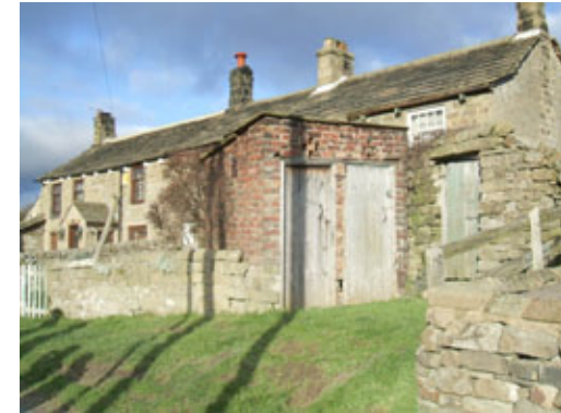
Stone terrace and brick privies at Valley View.
