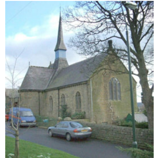
Converted Methodist Chapel opposite the green
