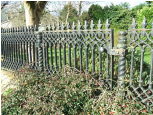
Railings on north side of Main Street.
