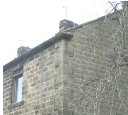
Quoins on West Cliff Terrace
