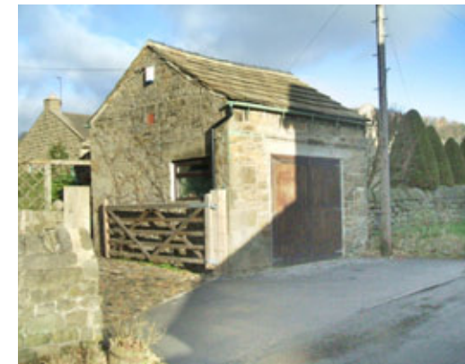
Stone slates on the roof of the former wet fish building.
