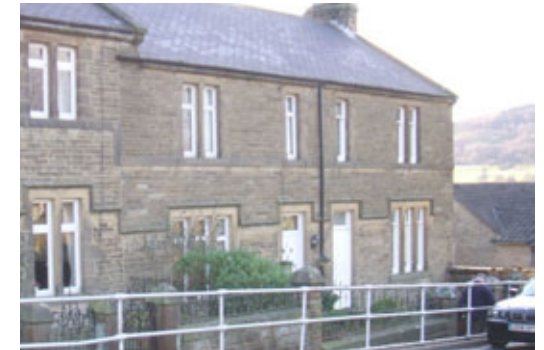
Mullion windows on Birch Field Terrace
