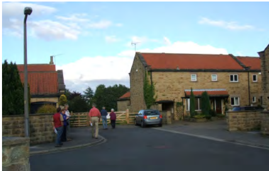
New development should respect the setting of the Conservation Area
