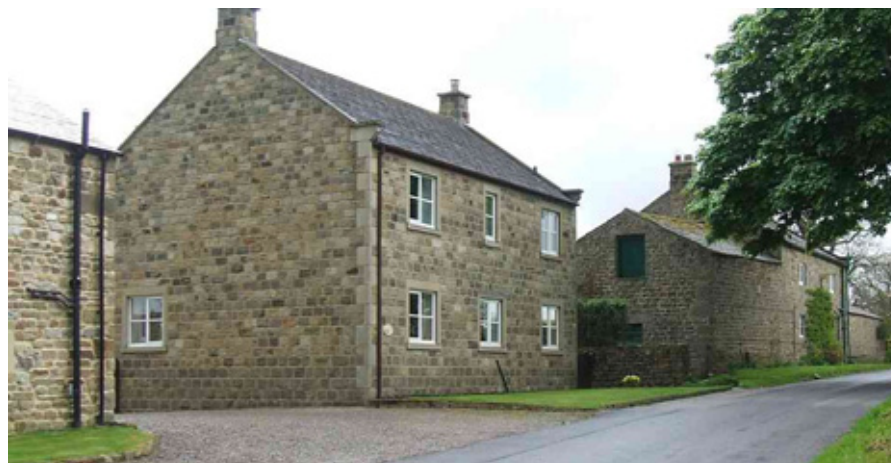
Sensitively designed new buildings, such as 'Greenacres' (above) can be integrated within the wider Conservation Area.
