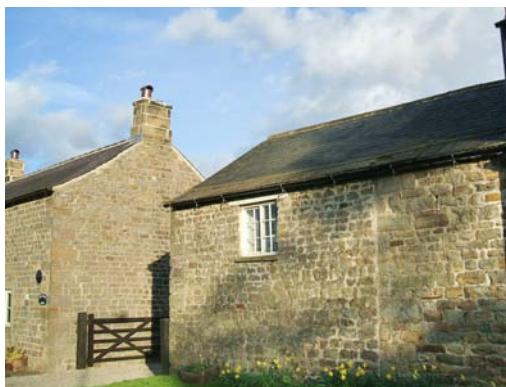
Low Moor Farm. The less important buildings on the right are faced with less regular stonework compared to the higher status farmhouse on the left
