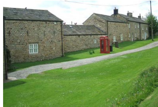
North vs. South: this pair of photographs illustrate the way building define the edges of the green and have eaves and ridges parallel to the street. Note how the south facing elevations have more windows and bigger windows than the north facing ones.
