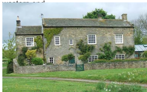
Holly Tree Farm. The change in stone suggests that the eaves were raised when the building was changed from thatch to stone slate.
