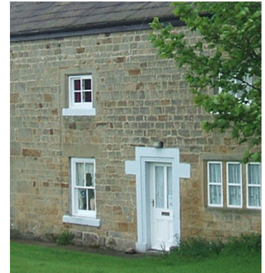
Chapel Farmhouse exhibits the three main window types in the village: mullioned casements (bottom right), Yorkshire sash (top left), and vertically sliding sash in a Victorian style opening (bottom left)
