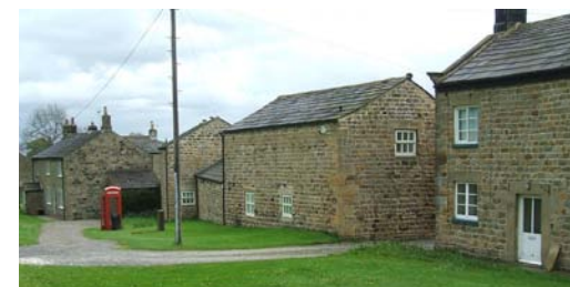
The cottages and former barns in the Chapel Farm group present an attractive, organic arrangement of masses to The Green. The buildings retain their traditional character.
