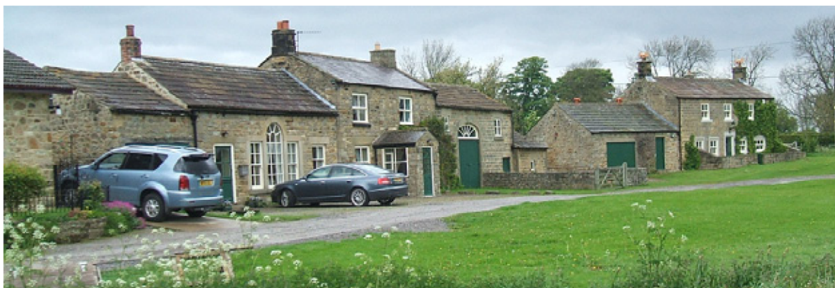
The organic layout of buildings with stepped eaves heights makes a positive contribution to the character and appearance of the Conservation Area.
