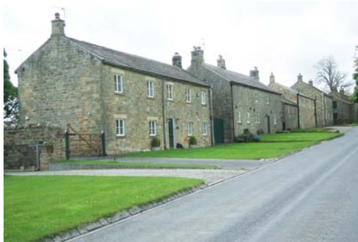
There is a consistent built form along the southern side of Fearby Road in this character area. Materials, chimneys and window details also help to unify the group
