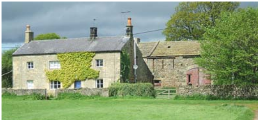
Manor House Farmhouse and its barn. The contrasting stonework of the house and barn is an attractive detail.
