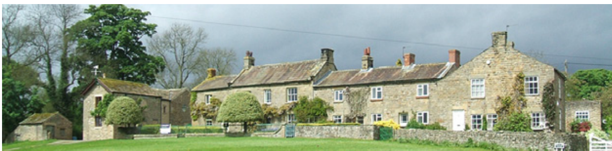
The Holly Tree House group (from left to right: former barn (now a house), principal house, and two ranges of former cottages)
