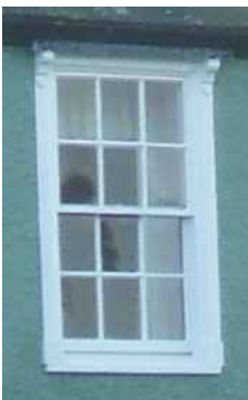
3) Tall multi-pane sash windows on a high status eighteenth century house.
