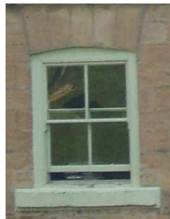
4) Larger paned sash typical of the later nineteenth century.
