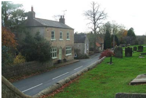
The elevated Churchyard gives Stang Lane a more open character, which is emphasised by the well spaced buildings across the lane. The Old Crown is shown here.
