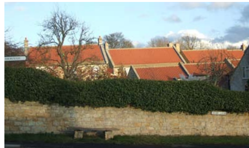
The tightly packed roofs of Manor Court.
