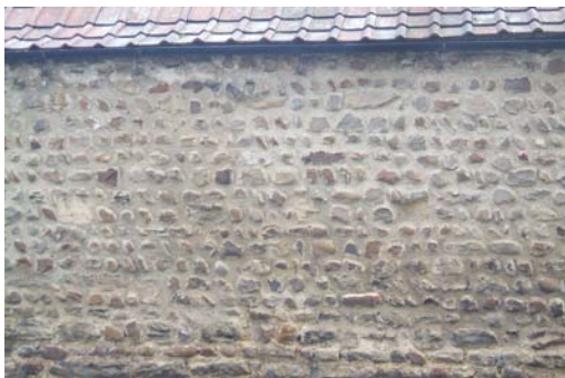
Coursed cobble walling at Garden Cottage.
