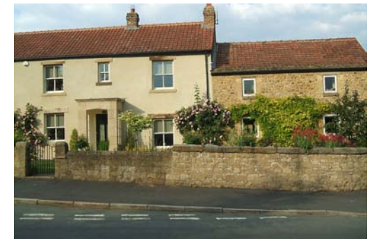
Manor Farm: the higher status farmhouse (left) is rendered to give the building an orderly, crisp appearance while the lower status barn (right) is faced with coursed rubble. These differences in status even continue to the treatment of the boundary walls.
