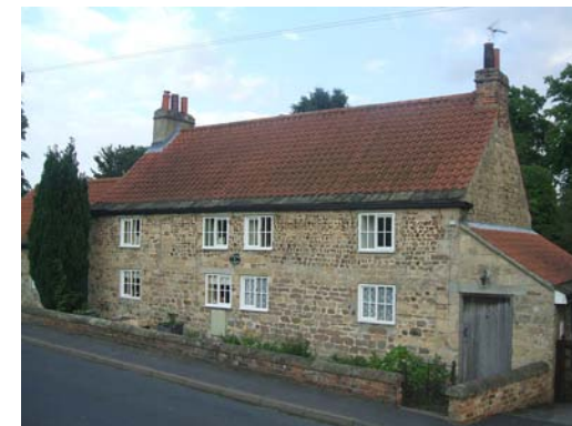
Coursed stone, coursed rubble, brick, cobble, render, pantiles, stone slates and timber. Most of the palette of traditional materials used in Farnham can be found on Lime Tree Cottages. These materials help to give a locally distinctive character.
