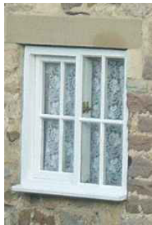
2) Sideways sliding Yorkshire sash windows in an eighteenth century cottage.
