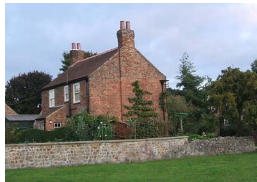
Pear Tree House, showing external chimney stack.
