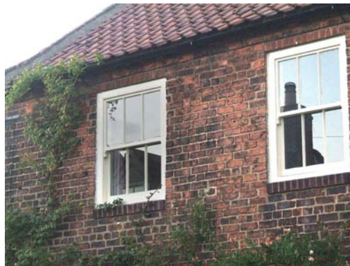
6 pane sliding sashes at Pear Tree House.
