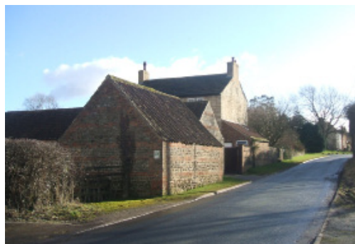
Cottage Farm from the north.
