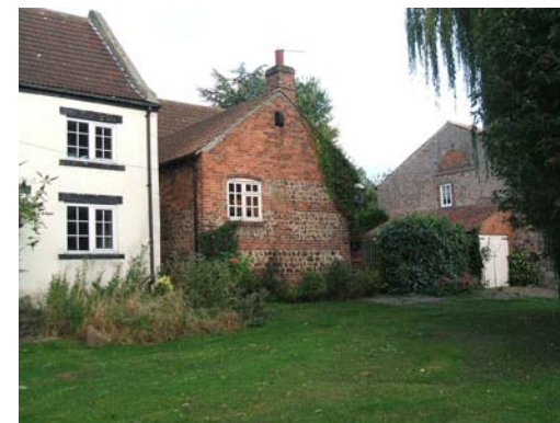
Ivy Cottage (left) and No. 8 Shortsill Lane (centre).
