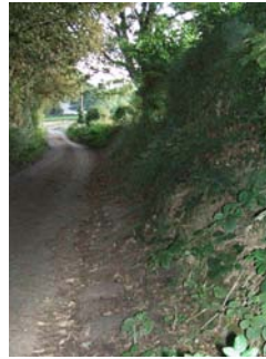
The enclosed stretch of Clifton Lane at the southern end of Clifton. The stone flags are visible in the foreground.
