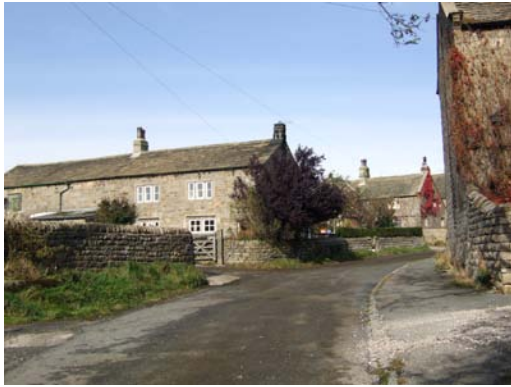
Wet and dry stone boundary walls make an important contribution to the character and appearance of Clifton
