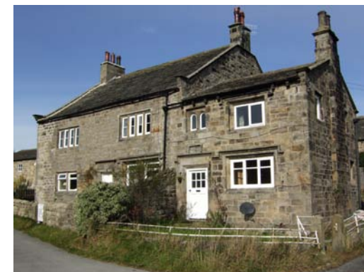
It appears that Fairfax Cottage (on right, dated 1604) was a large house which was part demolished to make way for Grange Farmhouse (dated 1728). The larger Grange Farmhouse incorporates one of the old window openings from the demolished part of Fairfax Cottage.
