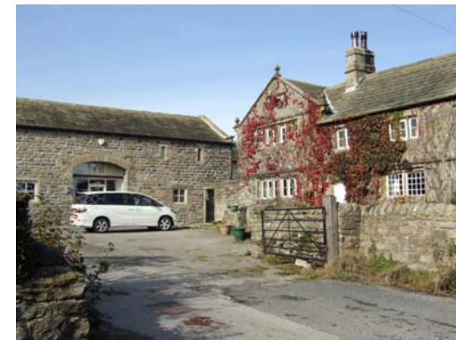
These very different buildings are unified by the use of local stone and stone slate for the roofs. The smooth stonework to Old Hall Farm differs significantly to the more roughly tooled stonework at Appletree Barn
