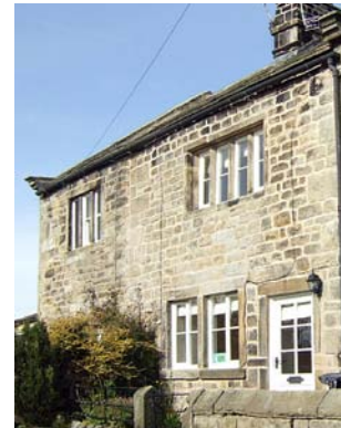
Clifton Cottage and Ash Tree Cottage exhibit the three principal window types in the Conservation Area: a seventeenth century opening with chamfered reveals and double chamfer mullions (top right), eighteenth century mullioned openings with squared reveals and square mullions (top left), and larger nineteenth century openings (bottom right).
