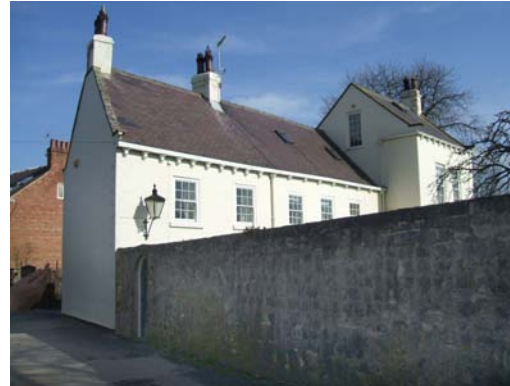
Vertical sliding sashes on Prospect House.
