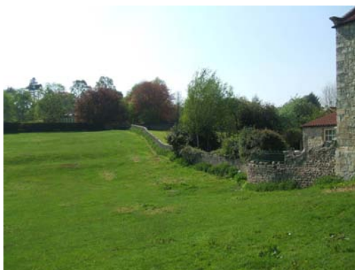
Limestone wall seen from Copgrove Road.
