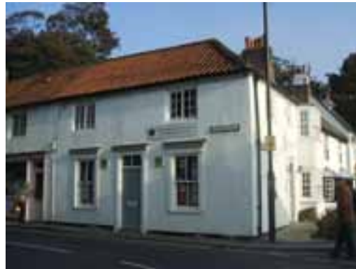
Yorkshire horizontal sliding sashes on the upper floor, vertical sliding sashes on the ground floor of this property on Fishergate
