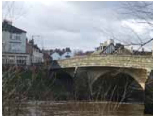
The bridge seen from the north bank of the river.
