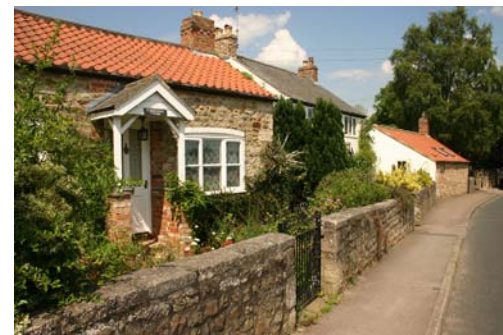
Cobblestone cottage with Yorkshire sliding sash.
