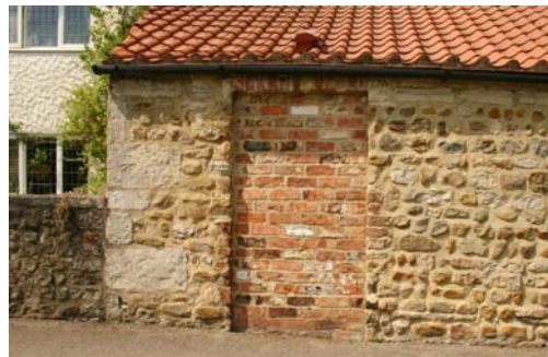
Cobble, brick, stone quoins and a pantile roof - defining materials in Bishopton.
