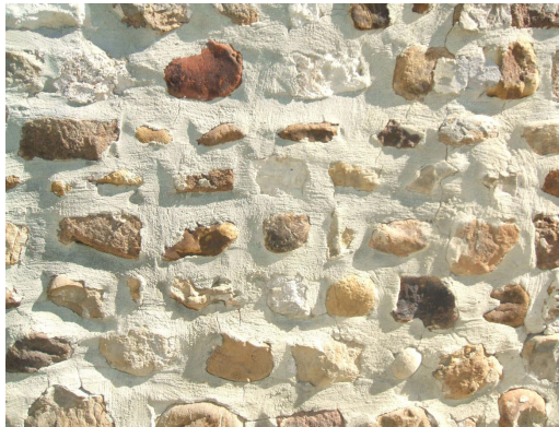
Field cobbles used in many lower status buildings and boundary walls within the village. Many of the buildings show evidence of being rendered over at some stage.
