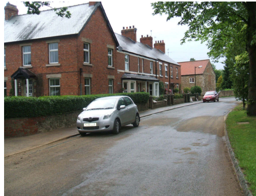
Fontein Terrace - a two storey brick terrace with a Welsh slate roof.
