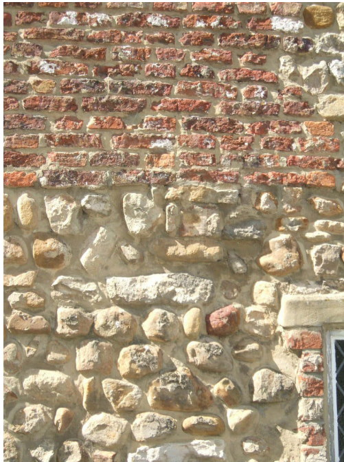
Soft clamped bricks mixed in this instance with a cobble infill.
