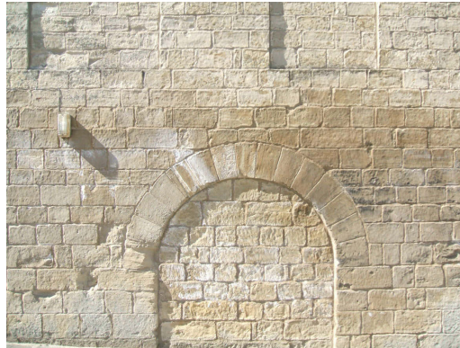
Coursed limestone walling.
