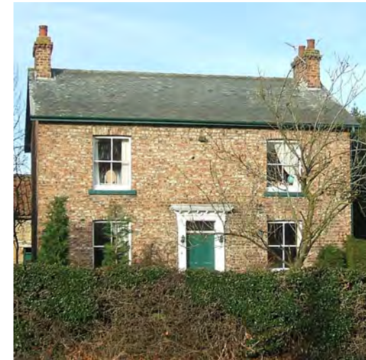
Ainsty Farm is constructed of traditional natural materials which are the most commonly used in the Conservation Area.
