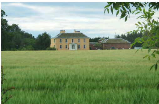
Bilton Hall. The later bay windows are just visible on the left, and the coach house is visible beyond the Hall.
