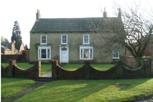
Chestnut House exhibits the grid-like layout of openings typically found on the larger houses in the conservation area. The roof detailing is also typical of the Conservation Area.
