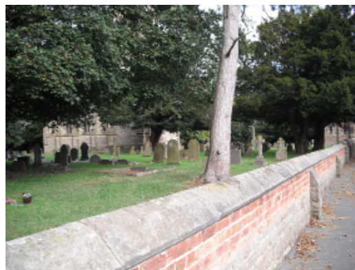
Church boundary wall.
