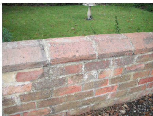
Cottage garden wall.
