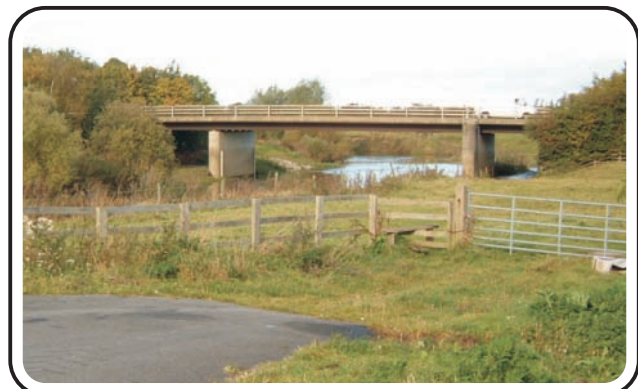
B Skip Bridge on the A59.
