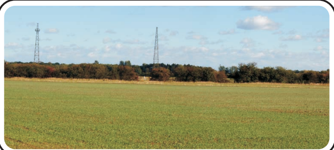
B Communications masts east of Norton-le-Clay.
