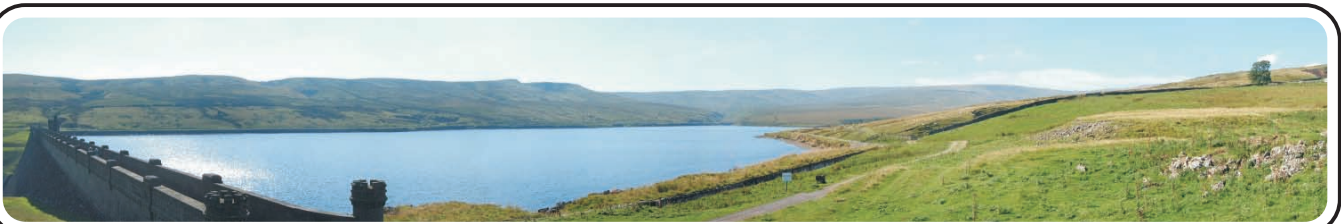
B Angram Reservoir and dam wall.
