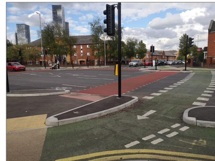
Figure 3.14. CYCLOPS signalised junction
