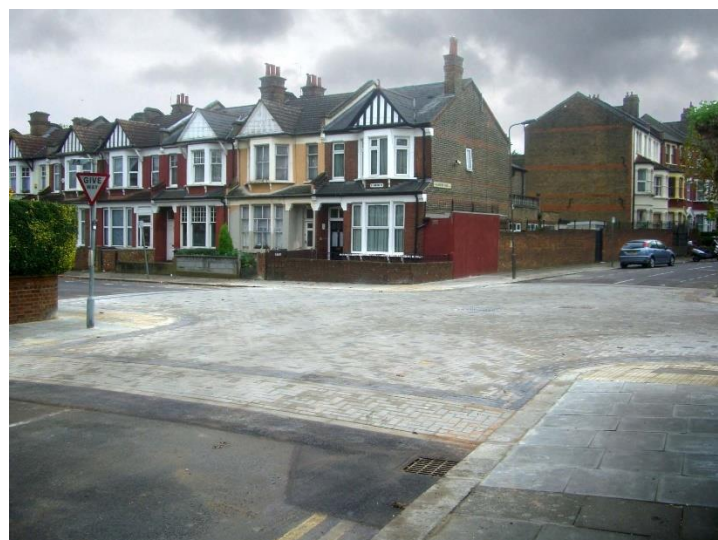
Figure 4.8. Raised table junction
