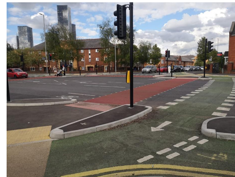
Figure 3.12. CYCLOPS signalised junction
