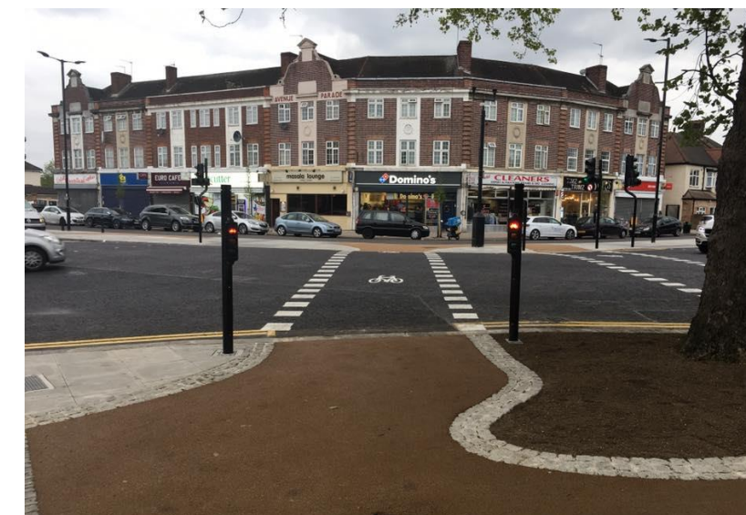
Figure 4.6. Improved signalised junction (Enfield)
