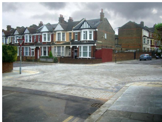
Figure 4.7. Raised table junction
