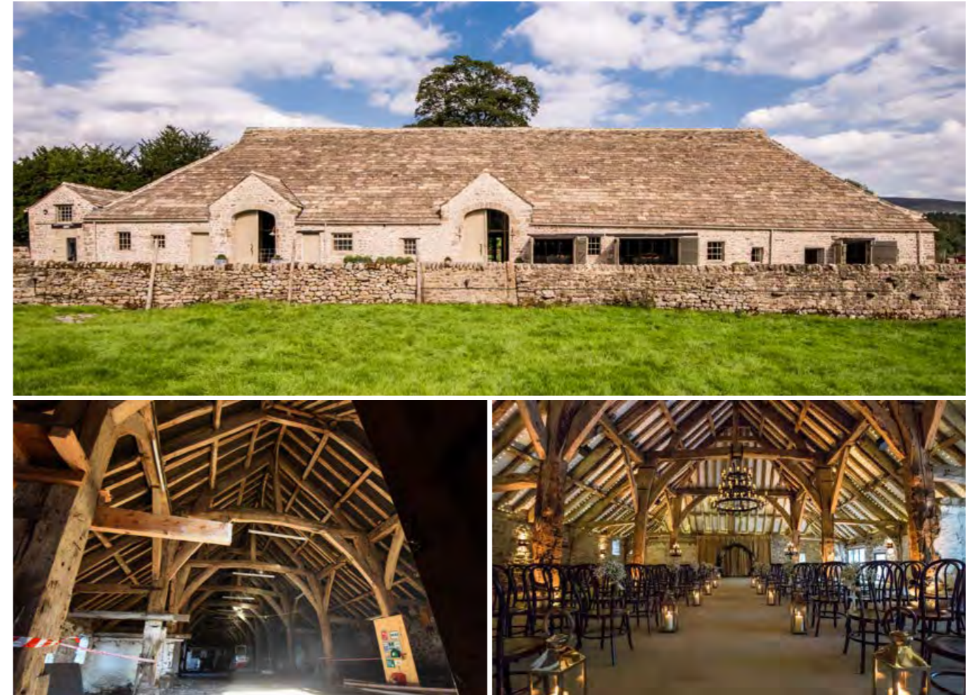
Top: Tithe Barn External Bottom-Left: Interior, Before Renovations Bottom-Right: Interior, After Renovations
