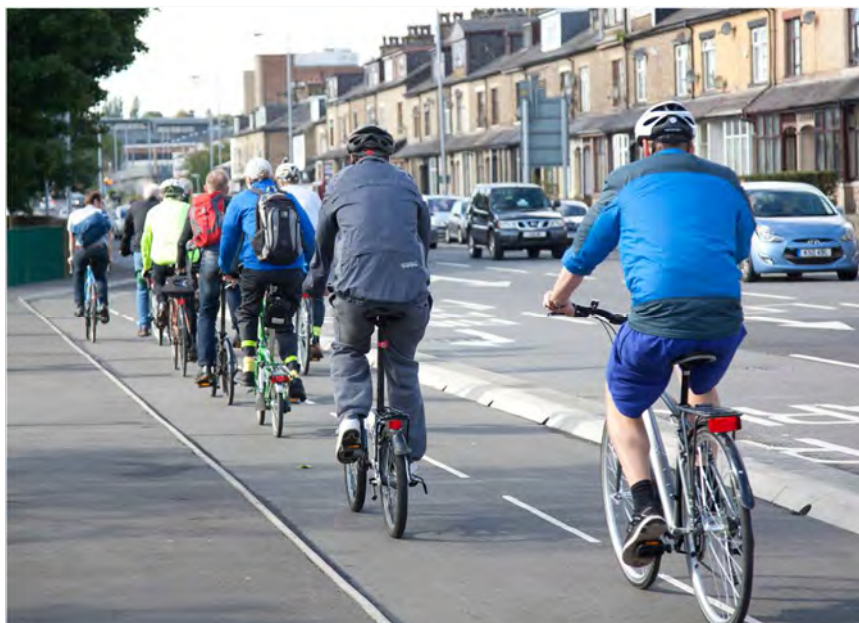
Figure 40 – Fully Segregated Two-Way Cycle Track (Leeds)
