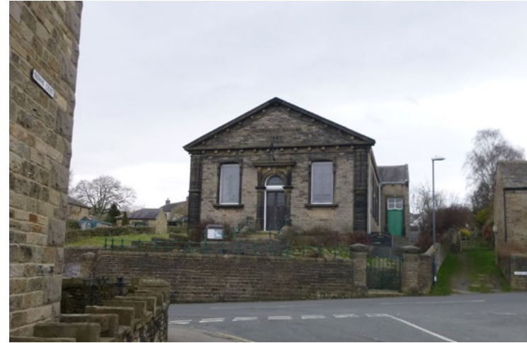
Methodist Church, Skipton Road
