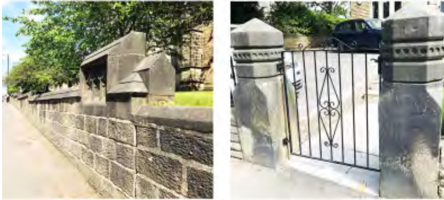
Figure 5.8 Traditional stone walling and gate piers in Harrogate
