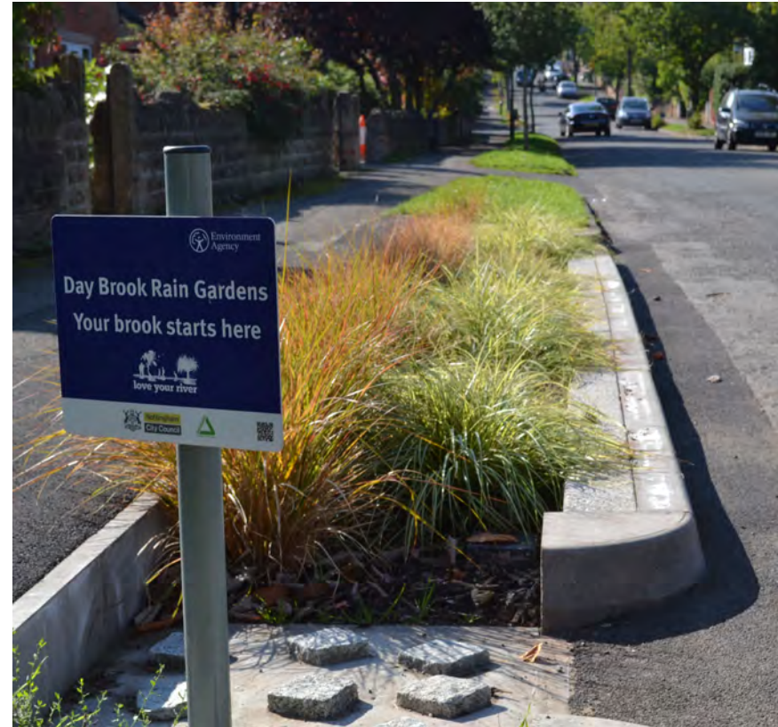
Figure 8.7 A Rain Garden on a Suburban Street
