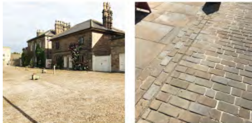
Figure 4.5 Examples of traditional materials used in pavements at Ripley and in Harrogate
