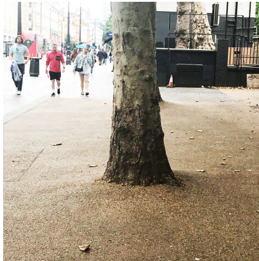
Figure 8.4 Porous wet pour rubber surface retrofitted around existing mature trees removes a trip hazard and allows rainwater to percolate to the roots
