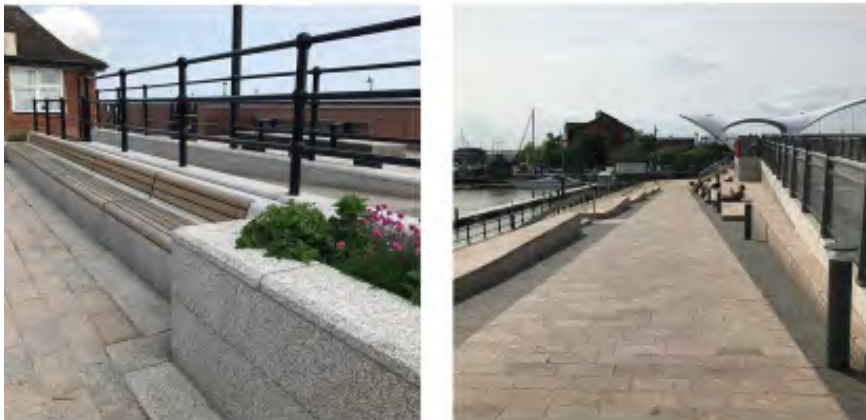
Figure 5.4 Seats Integrated into the Public Realm with Timber Slats and an example of Perching Places
