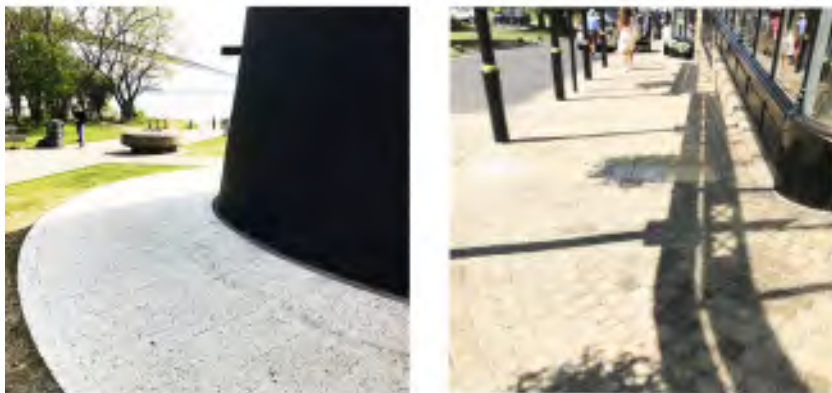
Figure 4.8 Examples of small paving units in Limestone and York stone laid to curves
