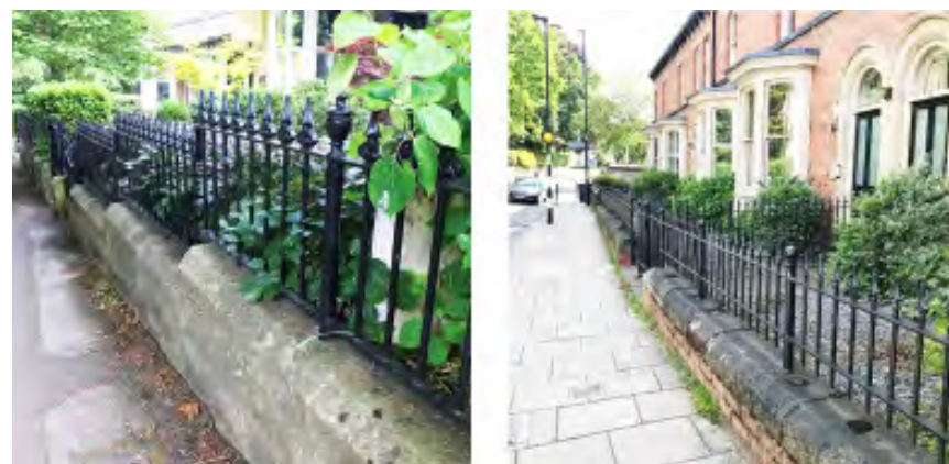
Figure 5.10 Examples of sympathetic replacement railings to domestic boundaries in Harrogate and Knaresborough
