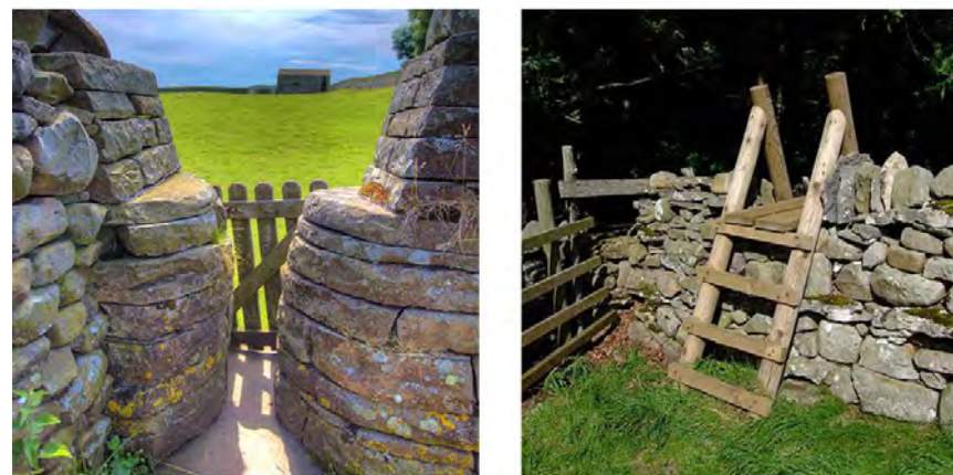
Figure 5.14 Traditional examples of stiles include a squeeze stile and a ladder stile
