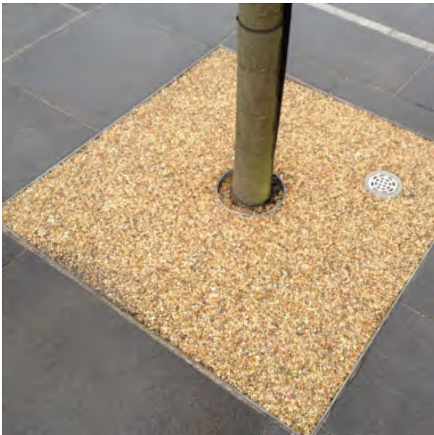
Figure 8.3 Porous resin bound gravel surfacing to tree pit of newly planted trees
