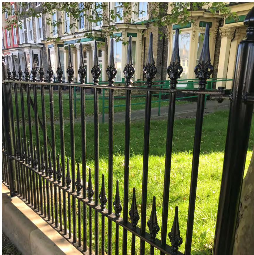
Figure 5.13 Note the changes in bar thickness and finial size between the leaf catcher and the main railing. This railing was informed with reference to historic photographs
