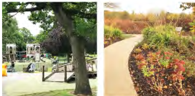
Figure 4.7 Examples of wet pour rubber surfacing in valley gardens and resin bound surfacing with aluminium edging
