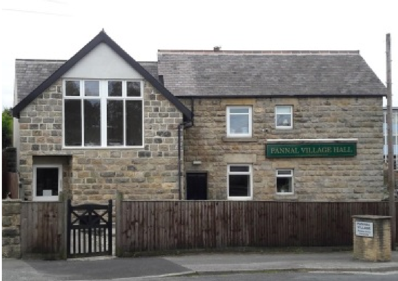
S106 monies have funded an extension to Pannal Village Hall and extensive internal improvements.
