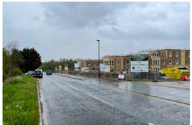
Existing footway/cycleway on Beckwith Head Road adjacent to H88.
