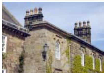
Well-designed, early 1990's extension to the Boar's Head.
