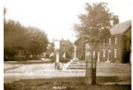
Looking towards the Castle Gatehouse.
