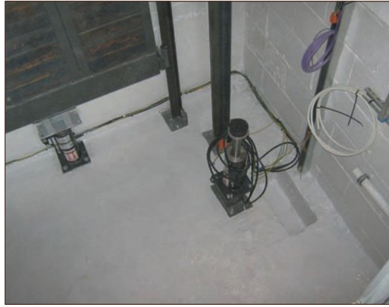
Figure A4.32 High quality installation of liquid gas membrane to lift pits, including resin gas protection on all screw penetrations (courtesy Card Geotechnics Limited)
