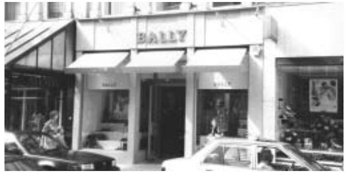
36 James Street, Harrogate: a simple, modern high quality shopfront with simple signage and well-integrated retractable awnings.
