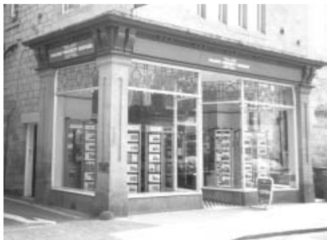
9 Albert Street, Harrogate: an unusual combination of stone piers and timber entablature.
