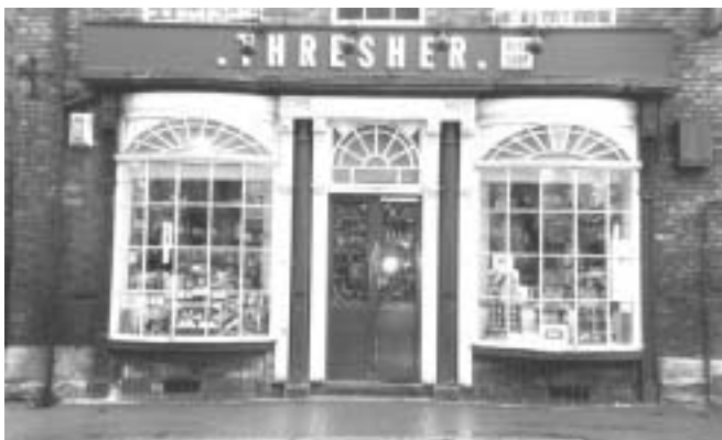
Georgian: small paned bow windows, slender pilasters and engaged columns
