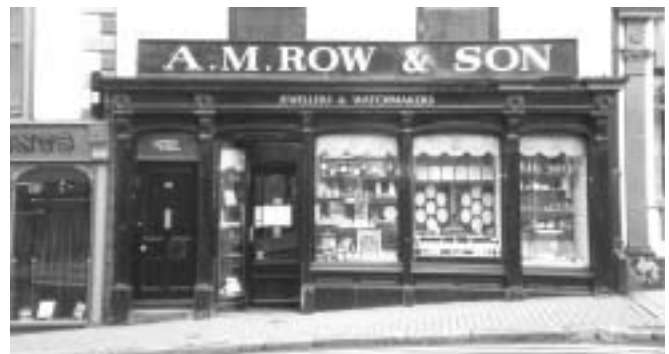
Victorian: full height panes divided by pilasters with consoles supporting the entablature
