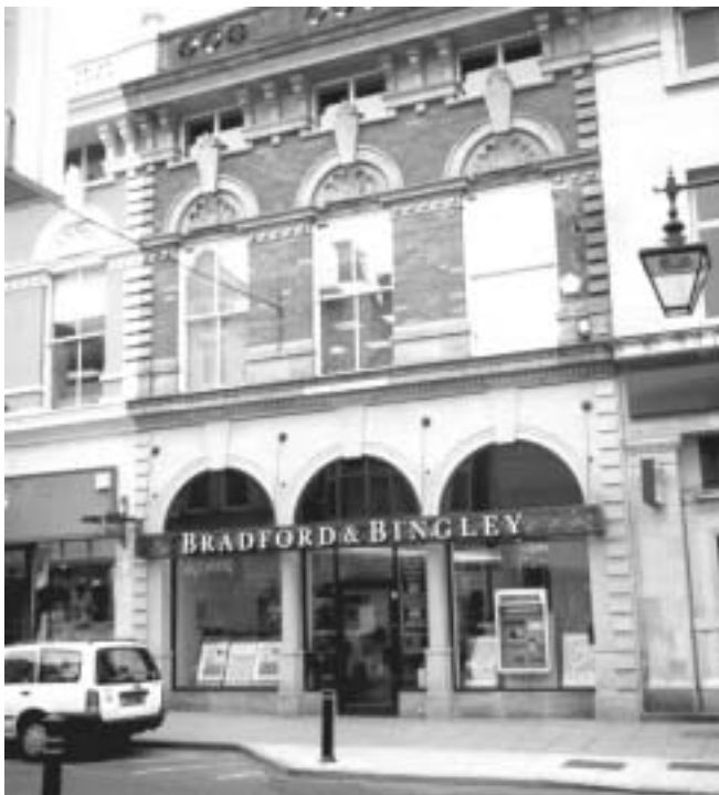
17 James Street, Harrogate: a high quality shopfront, well-related to the building & based on original arcading which extended along the Hirst Terrace.
