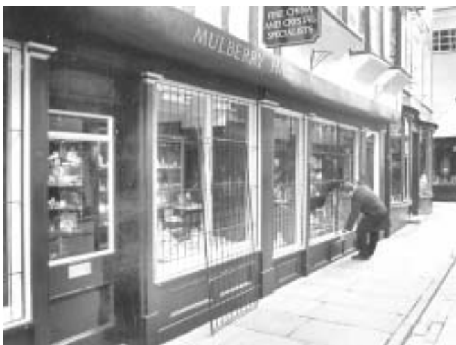
Open grilles maintain the interest of town centres and permit window shopping at night
