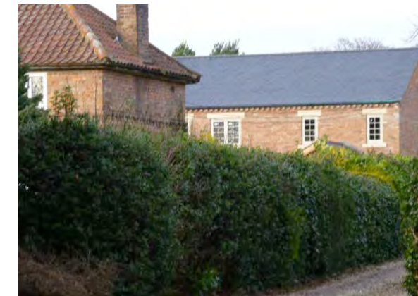
Unsuitable roofing material in Roecliffe Village
