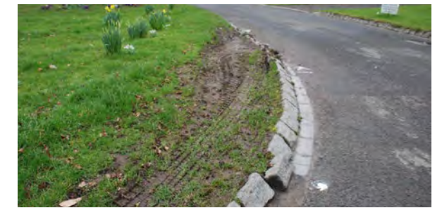
Damage to The Green opposite The Crown Inn
