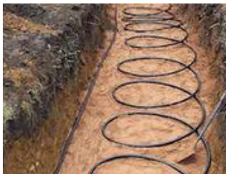
Ground source heat pumps
