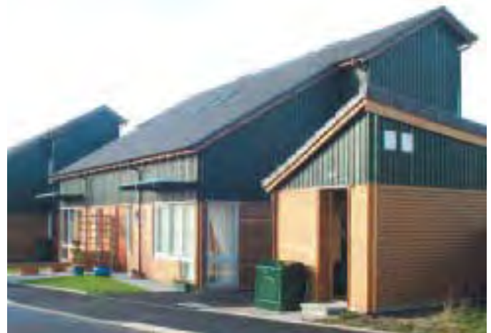
Figure 9 The energy centre for the Station Road district heating network in Newmachar, Scotland. It serves 14 semi-detached 2&3 bedroom houses and comprises a 12.5kWth, 5.5kWe Baxi DACHS CHP unit and two 38kW condensing gas-fired boilers. (Source: Community heating for planners and developers, Energy Saving Trust and Carbon Trust, December 2004)
