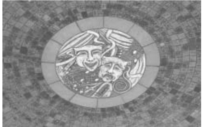
The theatrical themed roundel made of bronze, sandstone and granite sets on the road surface of Oxford Street Harrogate.
