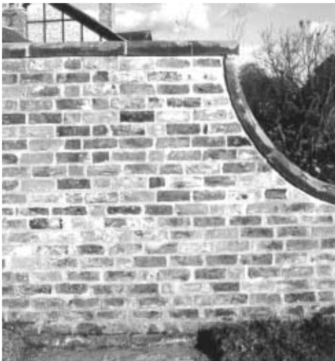
Brick wall at Kirk Hammerton
