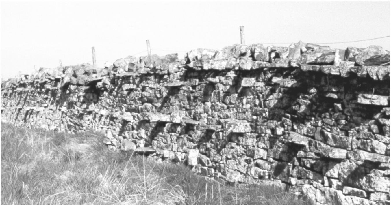
Masonry wall with square coping, Ripley Park.
