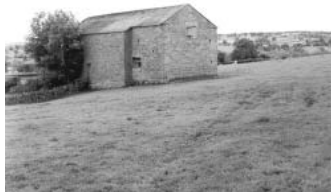
This barn sits comfortably in a wide open space and does not lend itself to conversion into a dwelling which would require the additional of a boundary wall.
