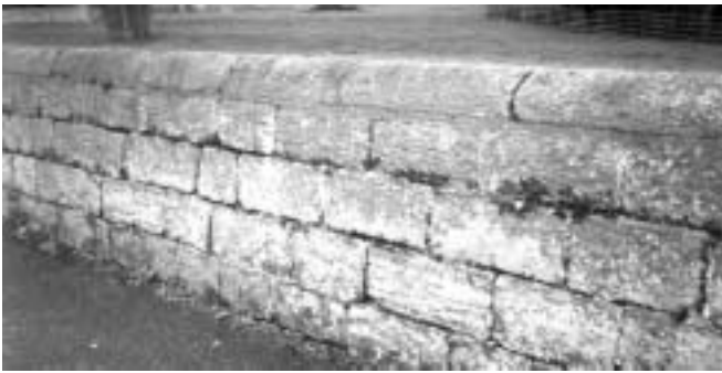
half-round copings on park wall at Killinghall.
