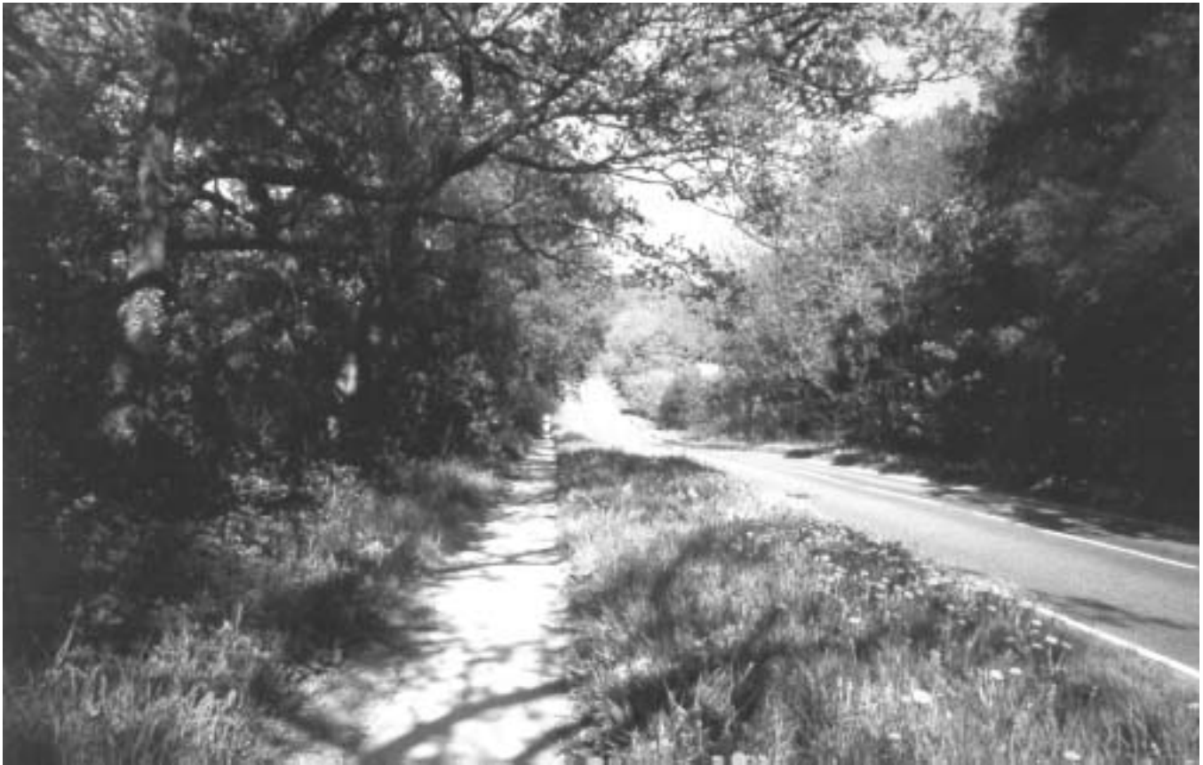
Footway separated from road by grass verge, Beckwithshaw.
