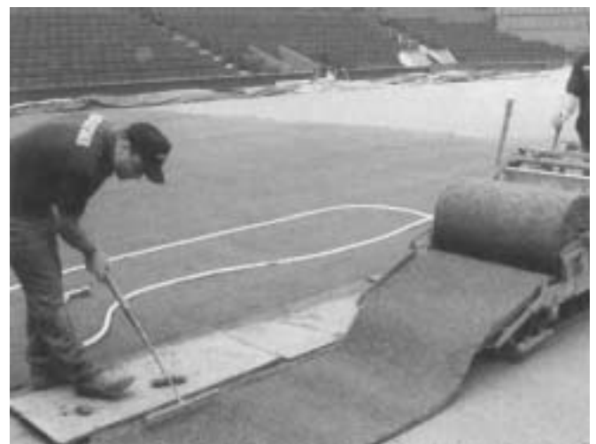
Sports pitch turf being laid.
