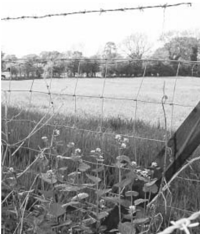
timber post and wire with lamb netting and barbed wire
