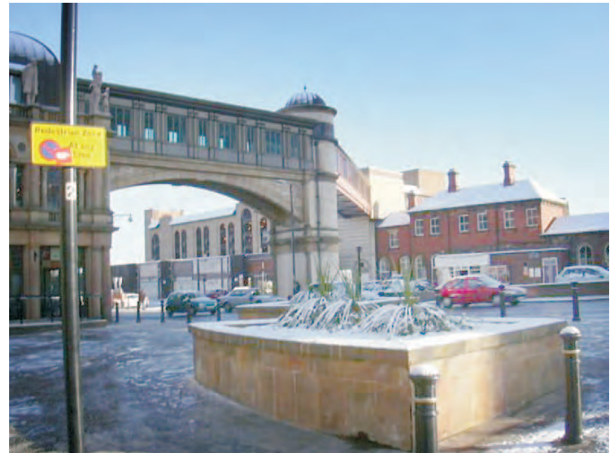
Station Parade - view of footbridge.
