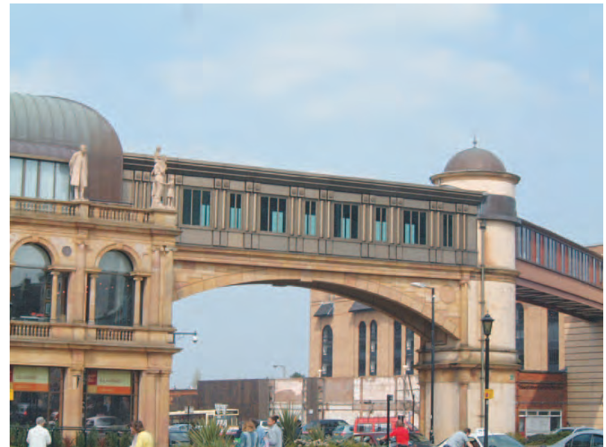
Bridge over Station Parade.
