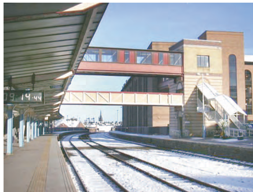
Station - view north to footbridge.
