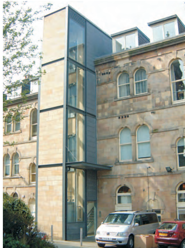
Ashlar infill to steel frame.
