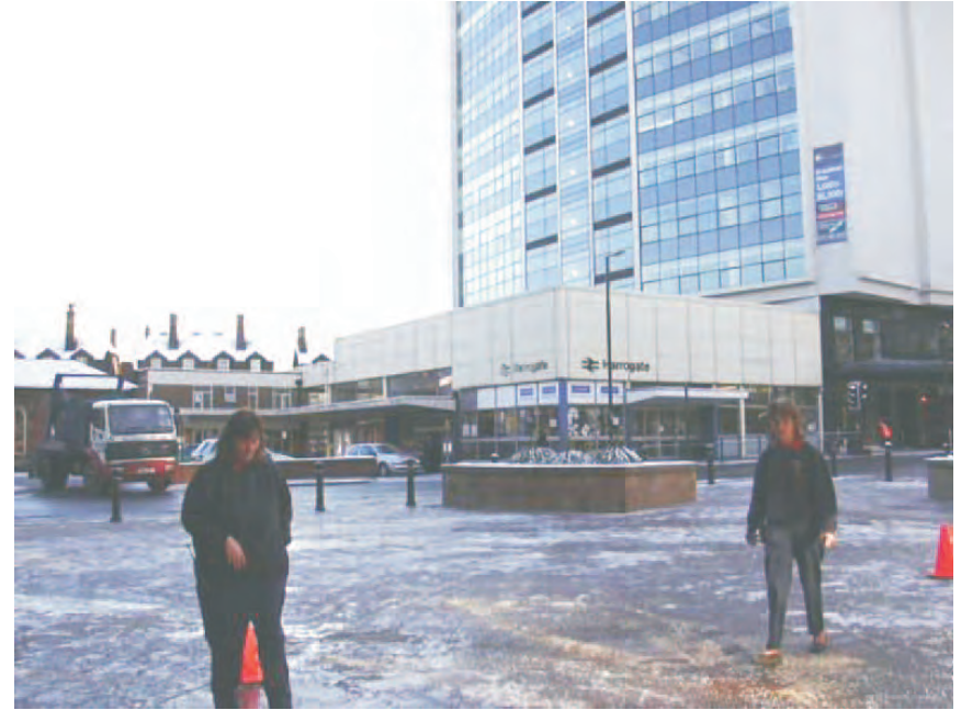
Station Parade - view of station.
