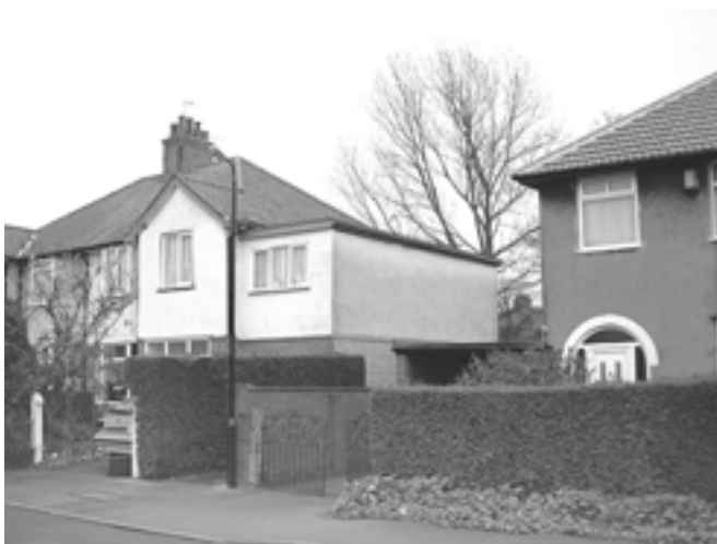
Prominent flat-roofed extension is visually detrimental.
