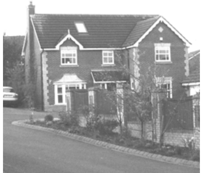
Two rooflights on opposite slopes of the roof resulting in an apparent 'hole' in the roof.
