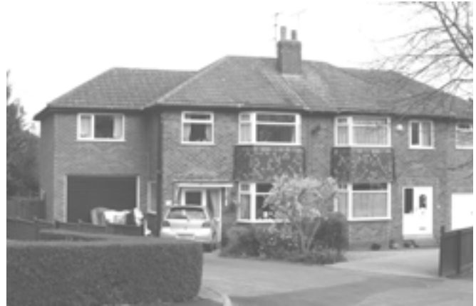
Extension set well back and reflecting the original form of the house.
