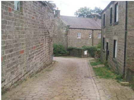
Robust gritstone buildings of Middlesmoor; two storey houses of rectangular plan form; unbroken dual pitched roofs finished in slate (Welsh or stone slate); chimneys at ridge ends; small window to wall ratio, deep set reveals to windows.
