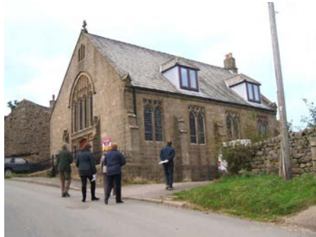
Chapel at Middlesmoor is of same materials as housing, but does not reflect same characteristics as the houses.
