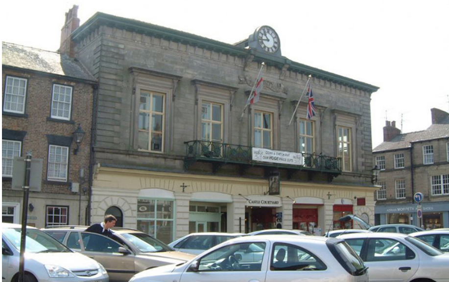
Highly decorative town hall in context of more modest stone and brick buildings.
