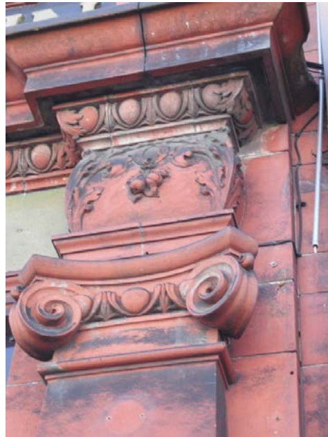
The decorative use of terracotta in the Starbeck Spa Conservation Area.
