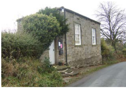
Leathley Chapel, grade II* listed, dating from 1826. Although a simple building, it displays a high degree of integrity, particularly internally where the original pews, surviving pulpit and communion rail still remain.
