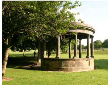
Tewit Well Cover, Harrogate. Dating from the beginning of the 19th century, this is a good example of a rare type of building, having been built specifically to cover the Tewit Well. The well was first discovered in 1571, the original cover having been replaced by this one, which was taken from the Old Sulphur Well when the Royal Pump Room was erected in 1842. It is grade II* listed which denotes it has a high degree of interest.
