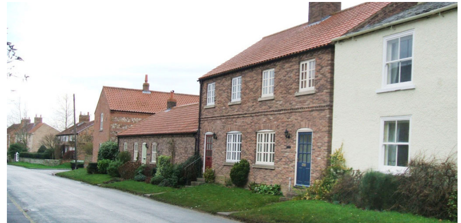
An example of a new dwelling demonstrating traditional, locally distinctive design in Great Ouseburn.
