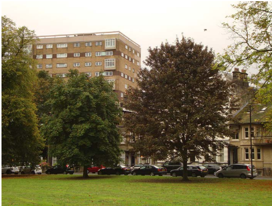
A 20th century apartment block, harmfully dominating the setting of the adjacent listed buildings.
