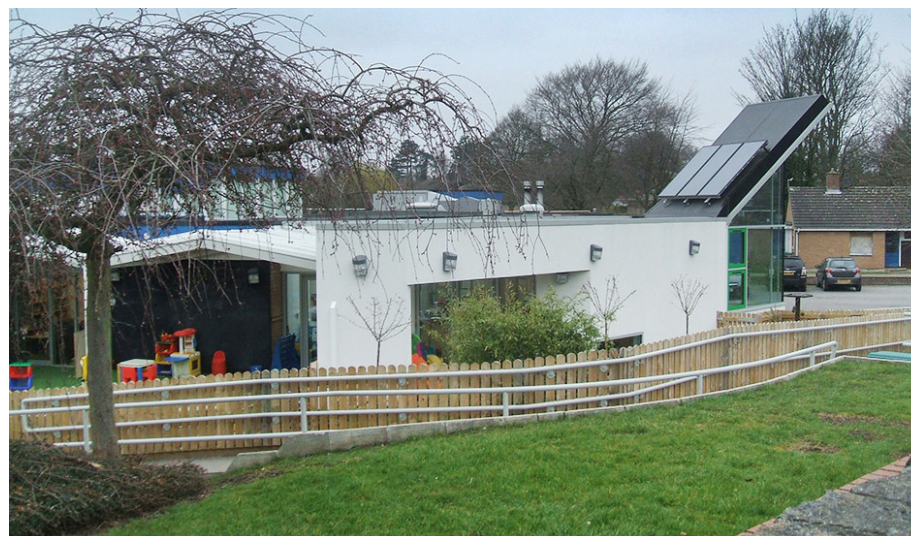
Solar panels on St Wilfrid’s Catholic Primary School, Ripon.
