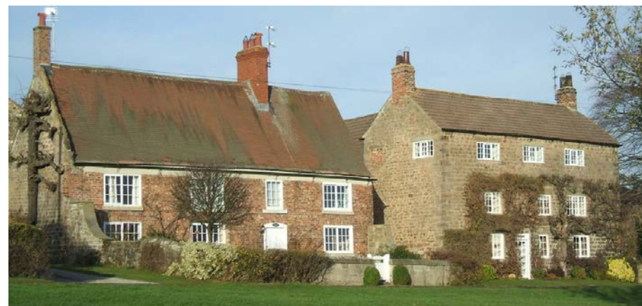
Traditional brick construction to left, note unusually steep roof.
