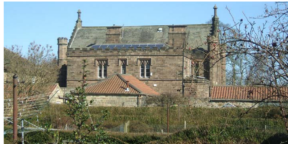
Solar panels partially hidden behind a parapet wall, Hotel de Ville, Ripley.
