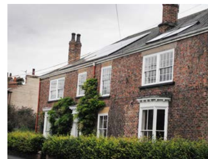
Visually prominent roof mounted solar panels, Main Street, Great Ouseburn.
