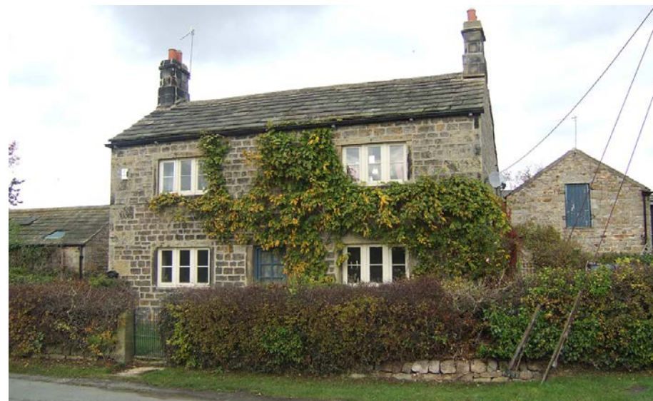
Traditional stone construction.
