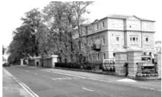
Queens Court, Harrogate - a car park redeveloped for office and residential use retained all the mature trees within the design.
