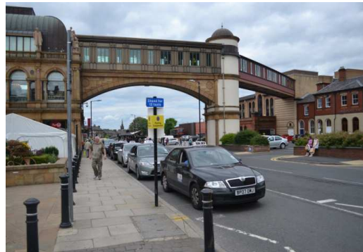
Bridge feature over Station Parade from Victoria Centre to Victoria Car Park
