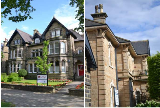
Victorian Style Villa/offices
